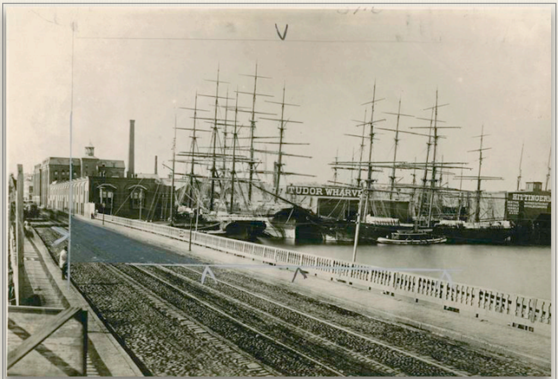
Charlestown Wharves – The Tudor Wharves are seen in the background.
