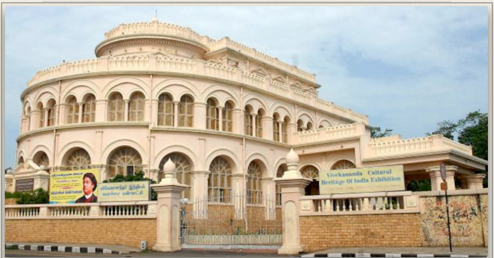
The Ice house in 2013. Windowed rooms used for living and work spaces were constructed around the outside of the well-insulated original cylinder. It now houses a museum of Vivekananda’s life and Indian culture.
